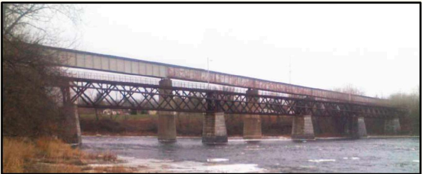
*fig. 6* Massena rail bridges crossing the Grasse River, truss bridge in foreground, girder bridge in background. Photo credit Russ Nelson<sup>5</sup>.
