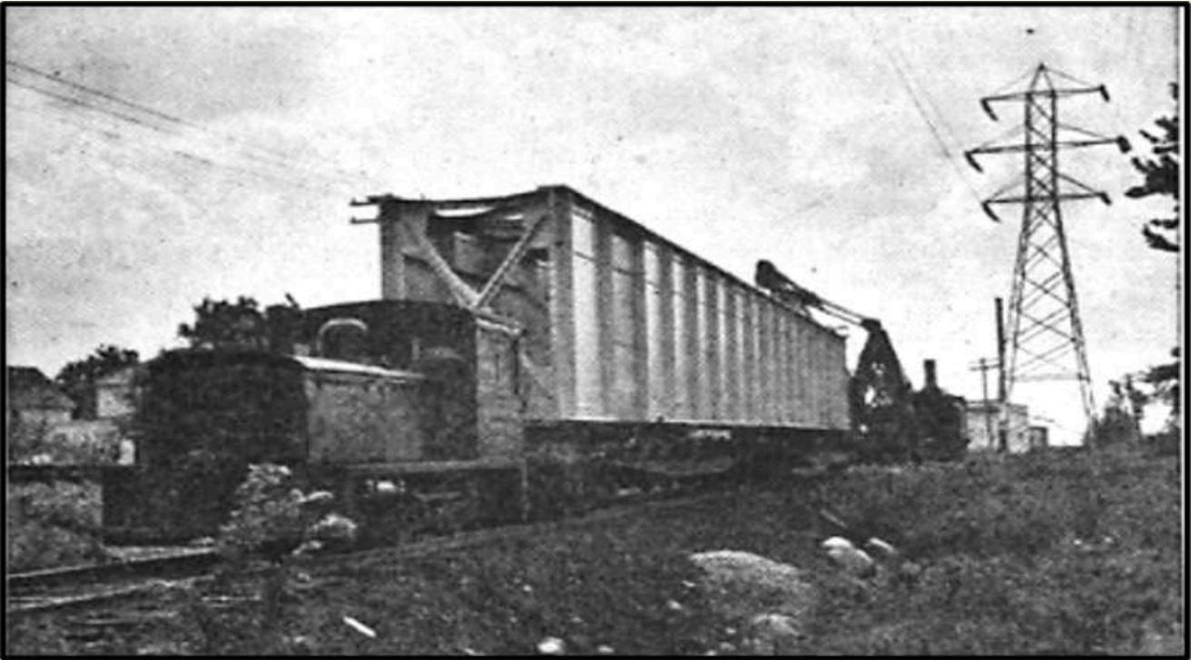
*fig. 8* Pre-assembled 100 foot, aluminium, deck plate-girder span being transported. Photo from *Railway Age*, All-Aluminum Bridge Span Makes Debut<sup>4</sup>.
