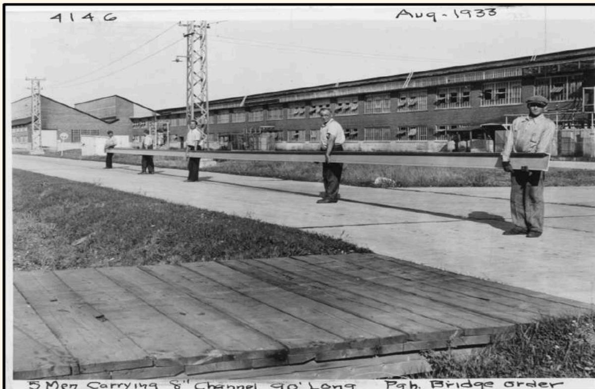
fig.5 Employees carrying a 27,4 meter (90 feet) section of 20 cm (8 inch) tall, U-shaped channel. Photo courtesy of NAPHA
