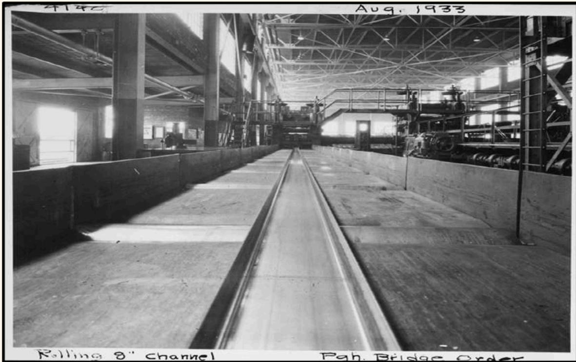
fig. 4 The Massena fabricating mill rolling sections that were over 27 meters in length with an aluminium channel at center of photo. Photo courtesy of NAPHA
